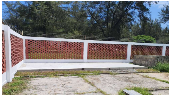
Foundation Construction (2 days)
