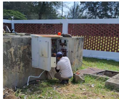
Electrical Construction Work (3 days)
